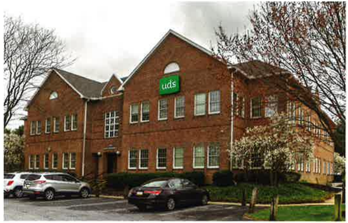
Caskey Group's professional installers recently installed signage throughout UDS's new location at Erin Court.
